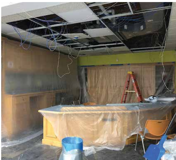
Work has begun to update the library's HVAC system.
