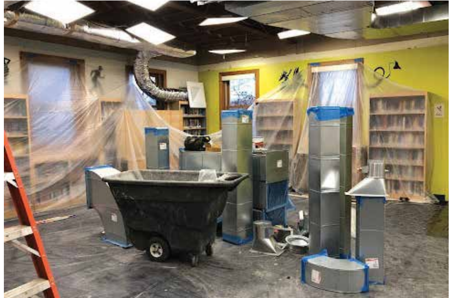
The Children's Room is under construction.
