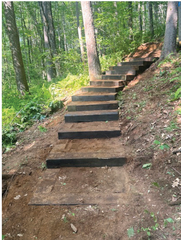
This photo shows the staircase halfway done.
