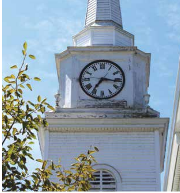
Paint is peeling and the clock face needs to be cleaned. TURLEY PHOTO BY PAULA OUIMETTE
