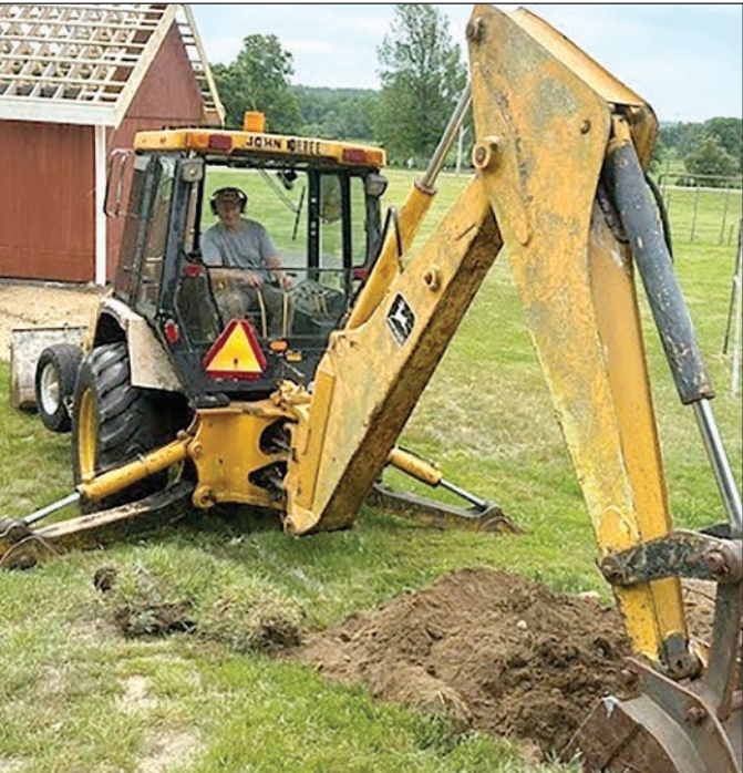
Jason Ayer operated his backhoe to dig the trench for the underground electric
