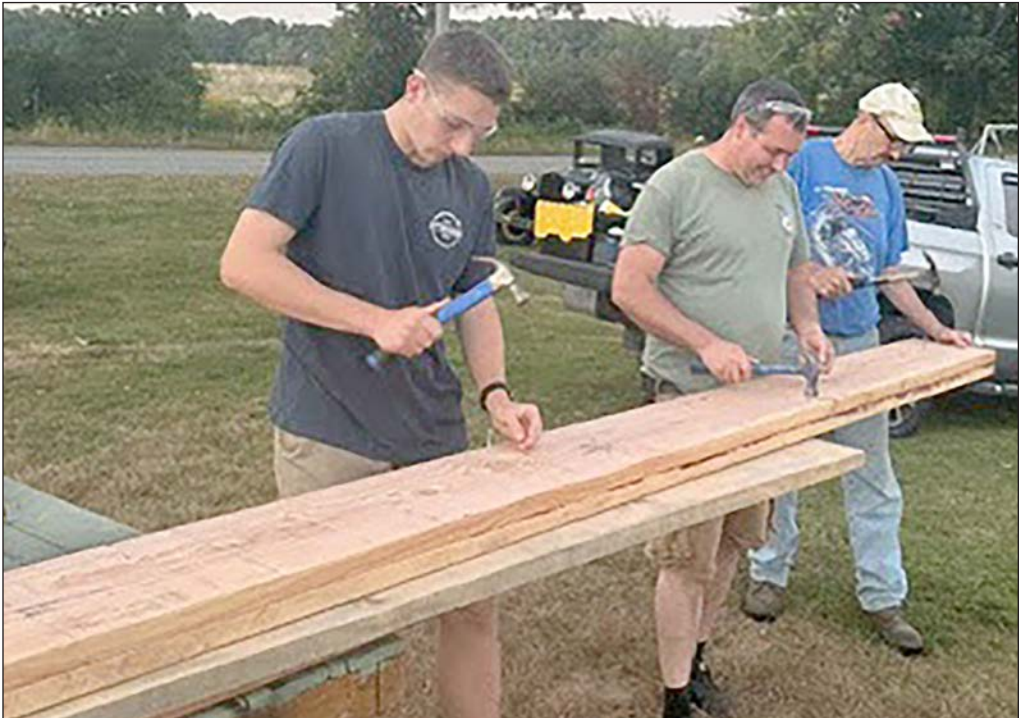
Ethan Salvatore, Dennis Letendre and John Head nailed boards together to create the beam to span the front opening of the pavilion.
