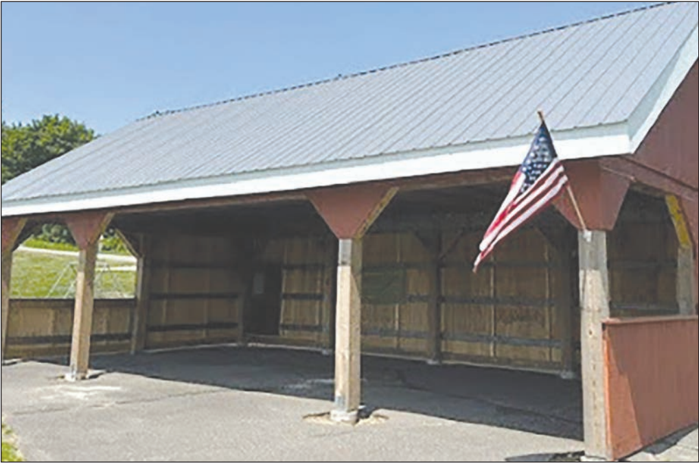
The completed New Braintree Pavilion.
