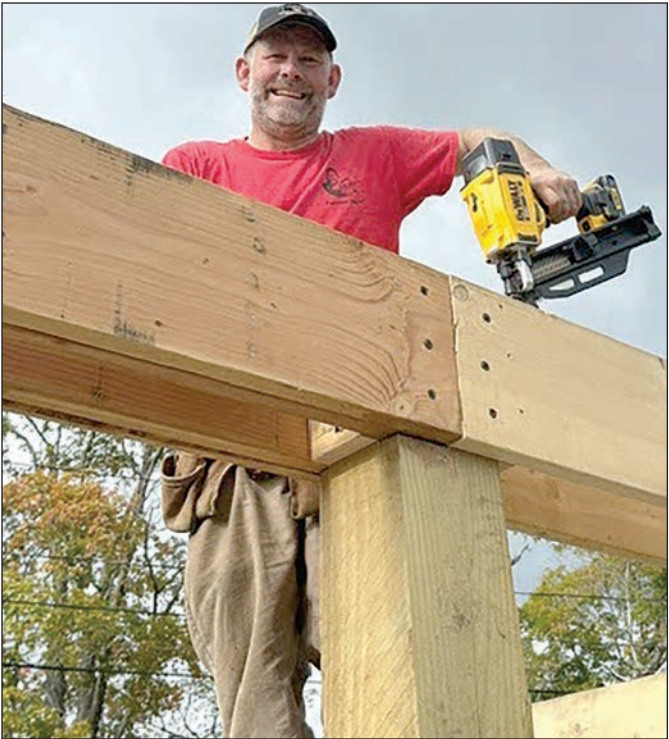
Matt Koziol attached the blocking brackets between the beams.
