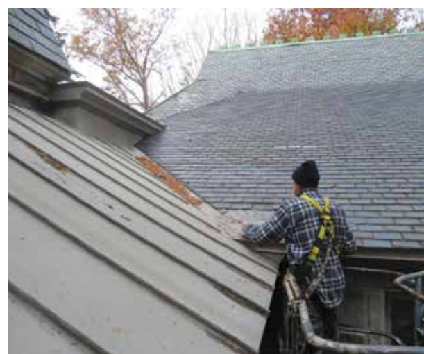
Skyline Engineers repair the Stone Church slate roof 2023.
